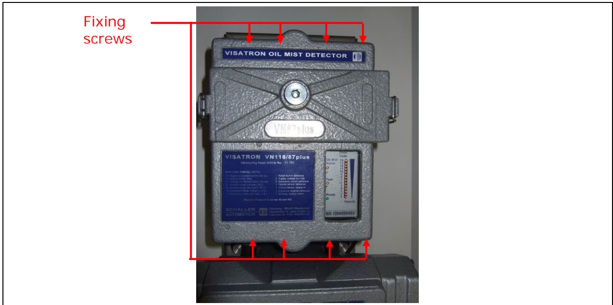
Figure 49: Step 3 is to unscrew the measuring head
