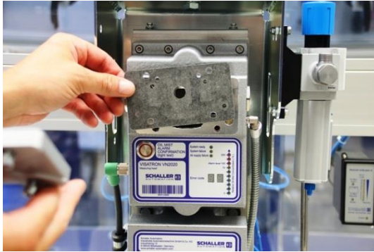
Figure 144: Remove the inspection cover seal
