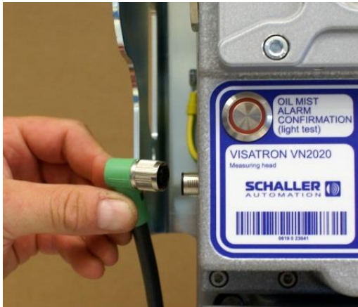
Figure 104: Unplug plug-in connector
