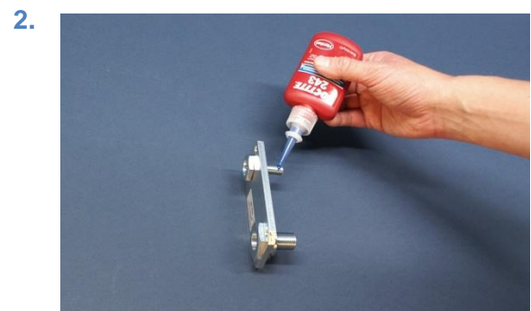
Figure 24: Screws with Loctite
