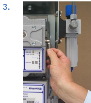
Figure 156: mounting compressed air hose
