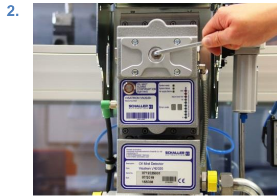
Figure 181: Inspection cover with mounted quick coupling cover
