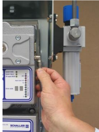
Figure 176: mounting of compressed air hose
