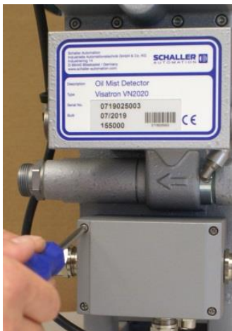
Figure 142: mounting of cover
