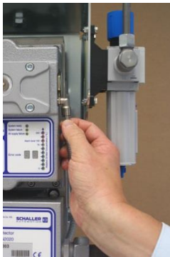
Figure 120: mounting of compressed air hose
