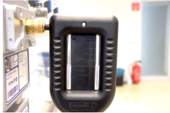
Figure 59: Negative pressure display on the U-tube manometer
