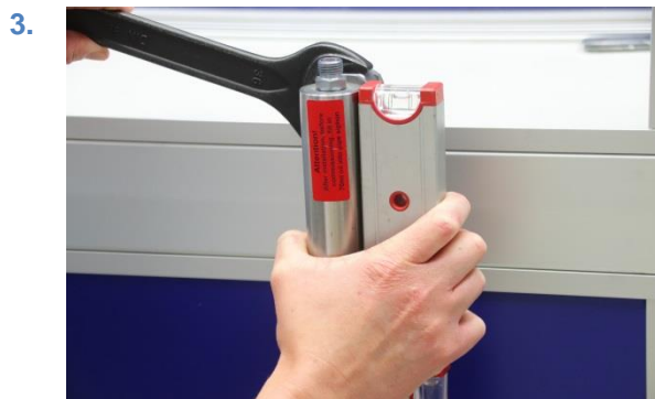
Figure 38: level of pipe siphon
